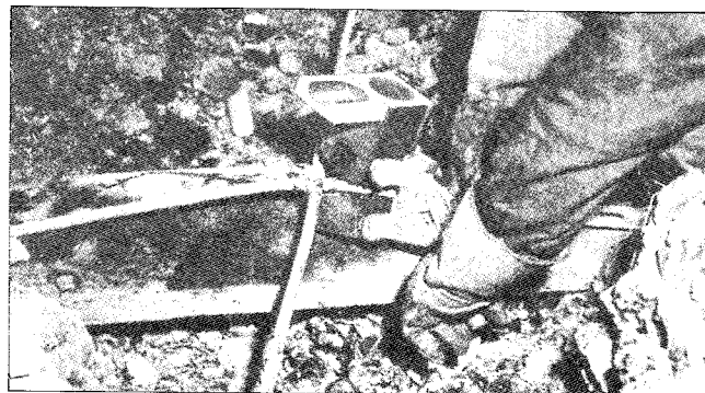
Removal of the mold exposes a CC4 cross connection
